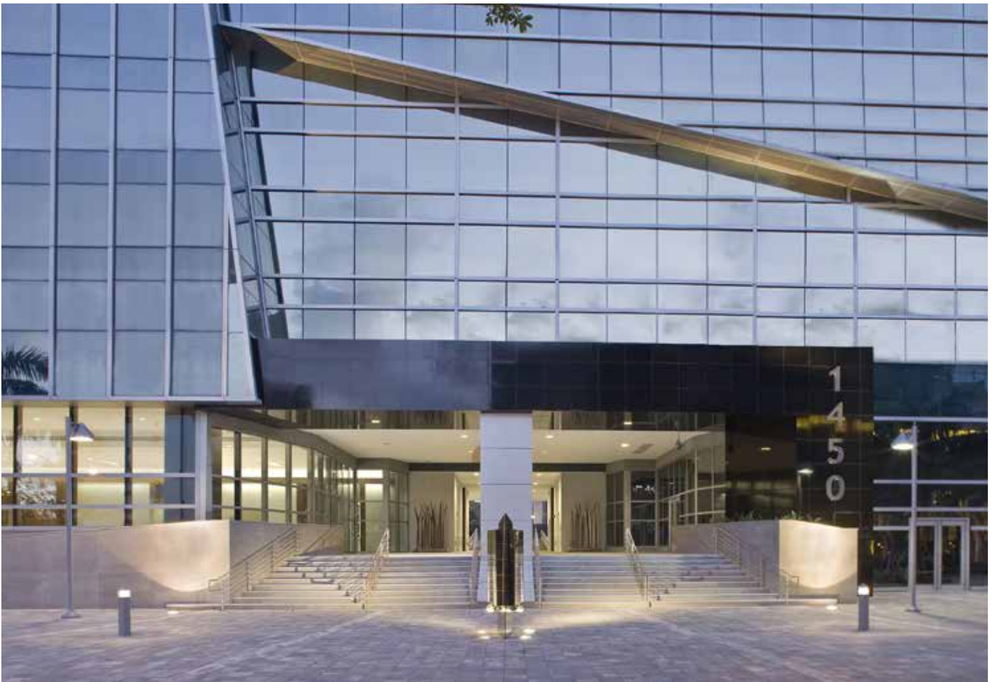
The Brickell Avenue entrance, with the breezeway straight ahead and the main lobby on the left. The lobby is raised several feet above the street level and the floodplain.
