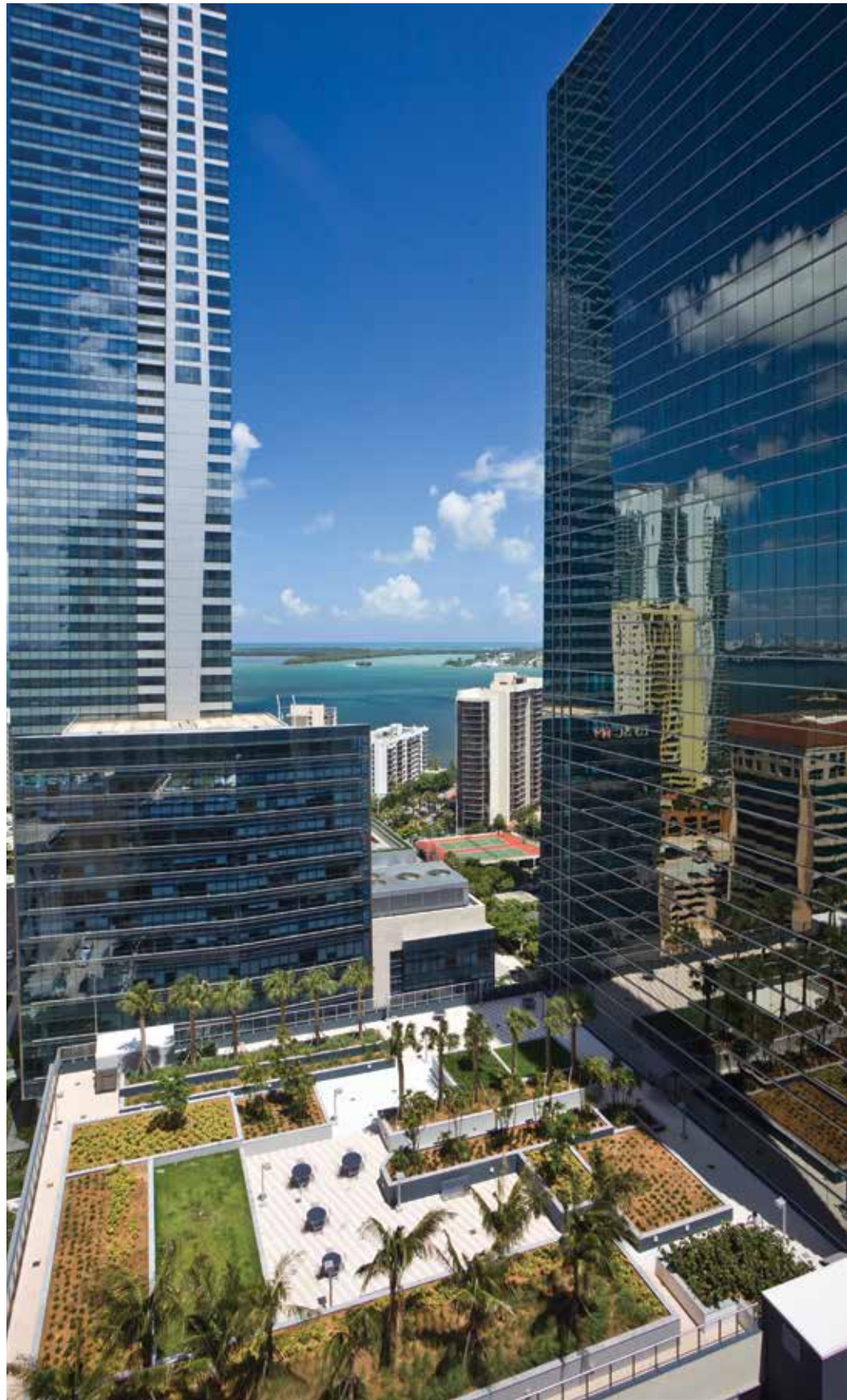
A rooftop garden on the 14th floor is located above the 13-story parking garage and offers views of Biscayne Bay and the surrounding Brickell district.
