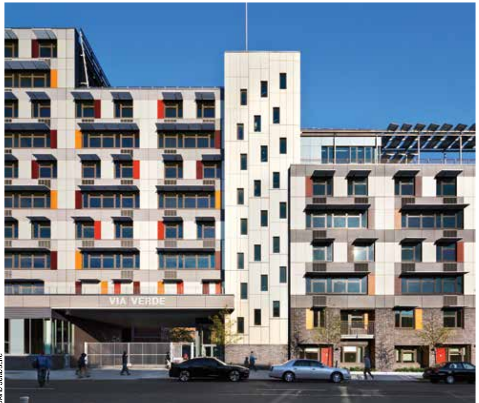
Windows along all stairwells provide daylight to encourage residents to take the stairs. The building exterior is a highly insulated modular system. Sunshades add interest and reduce use of air conditioning.
