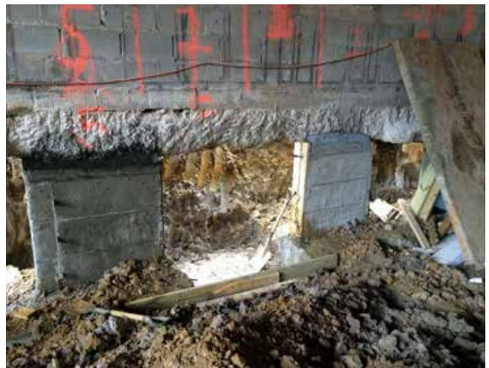
The original foundation was retained but required underpinning to allow for the creation of a new lower level.
