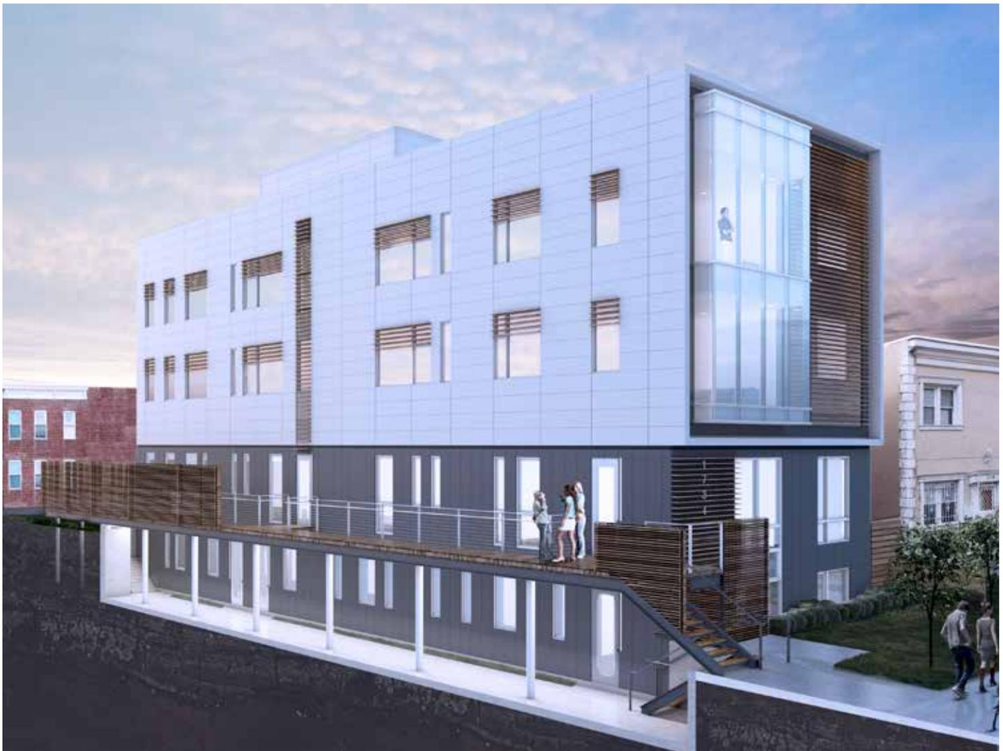
A rendering of the building highlights the cellar level, the floating entry bridge on the second level, and the upper levels sheathed in fiber-cement board.
