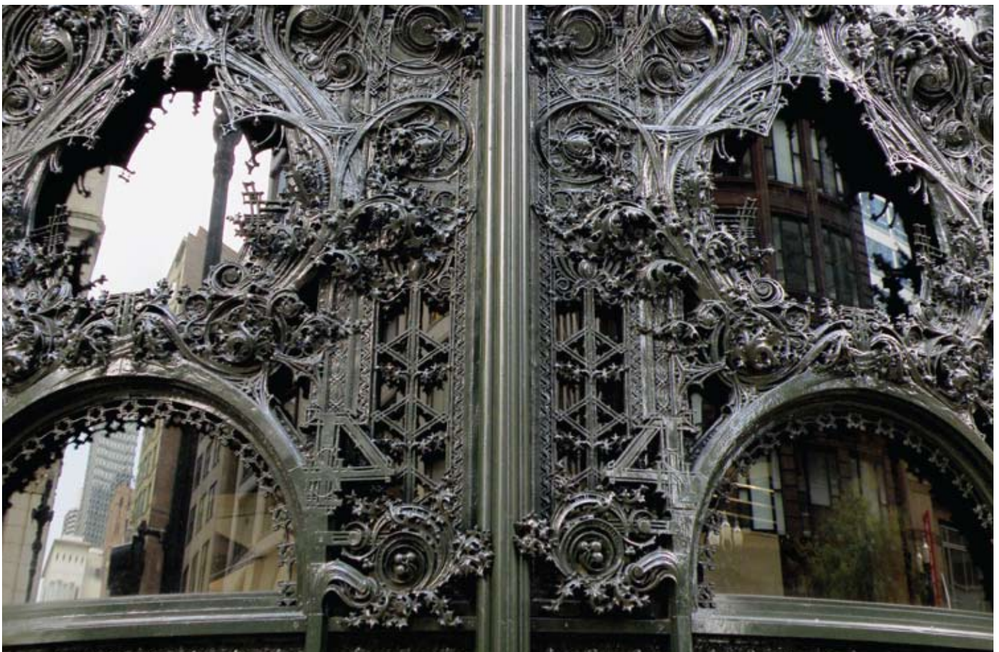
A close-up view of the cast ironwork on the rotunda after restoration.
