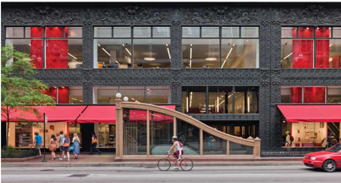
The historic cast ironwork along the State Street facade had deteriorated. Restoration involved documenting each piece, removing it, restoring it, then reattaching it to the building.
