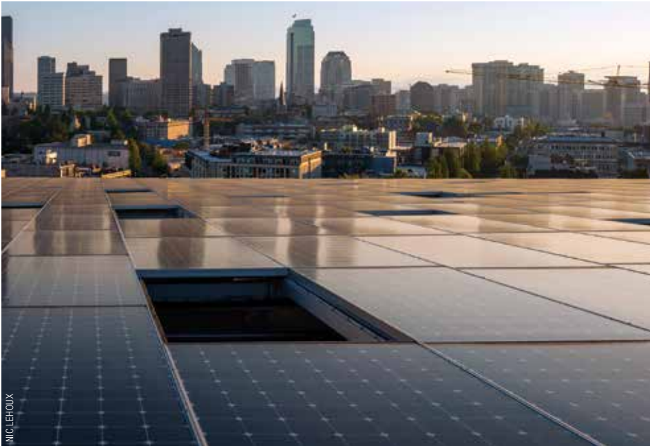
The Bullitt Center's 14,000-square-foot photovoltaic array on the roof comprises 575 modules with a peak generating capacity of 242 kilowatts (kW). In 2014, the building produced 243,761 kilowatt-hours (kWh) but consumed only 152,878 kWh.
