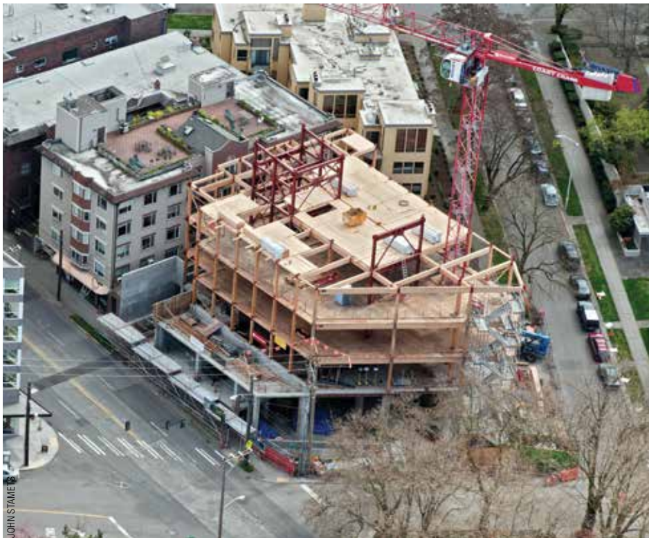
The building during construction, highlighting the combination of concrete and heavy-timber framing used in the structure.
