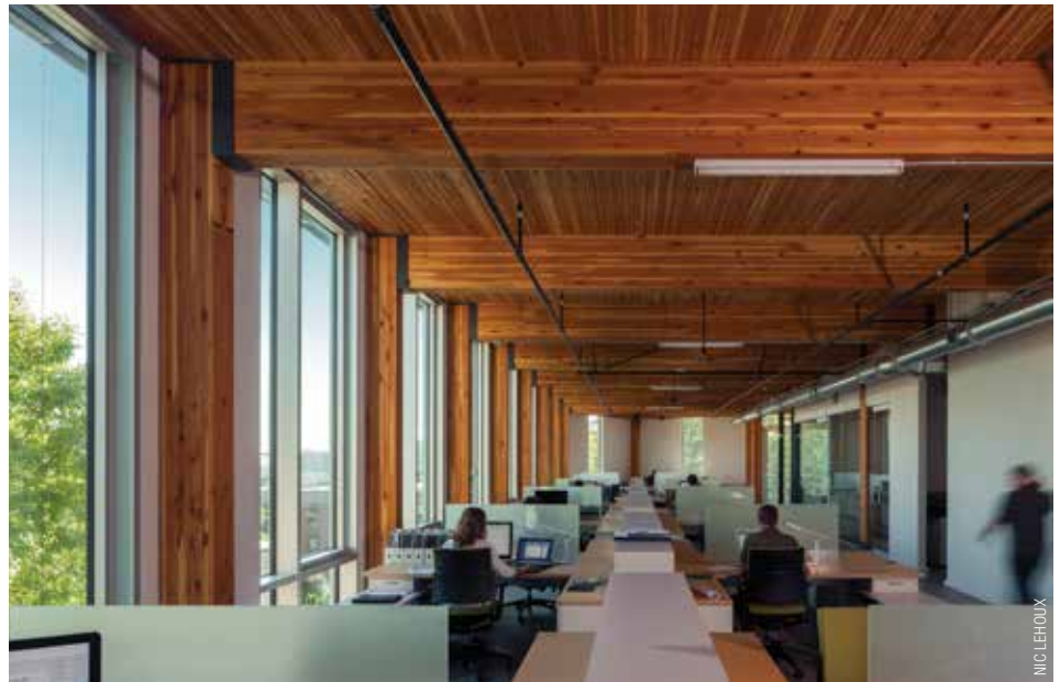
The use of heavy timber in the building's construction provides a strong aesthetic element for the interior while minimizing carbon-dioxide emissions that are the result of traditional concrete construction, and also serving as a carbon sink. In addition, every piece of wood in the structure has been certified by the Forest Stewardship Council.
