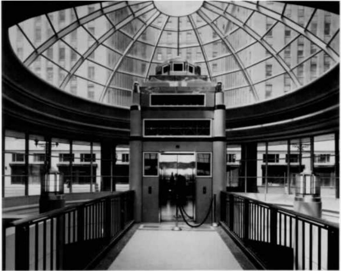
Interior of the Prospect Avenue entrance, featuring a domed skylight and elevator/escalator access to the lower level retail and transit areas.
