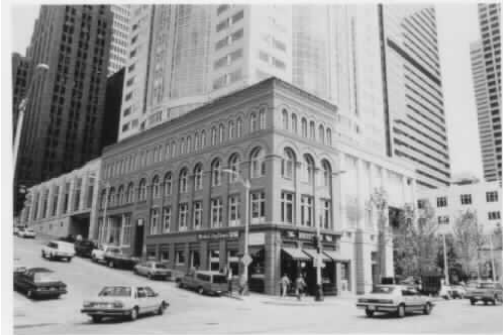
The facade of the historic Brooklyn Building was preserved, and the structure was incorporated into the base of the tower complex.
