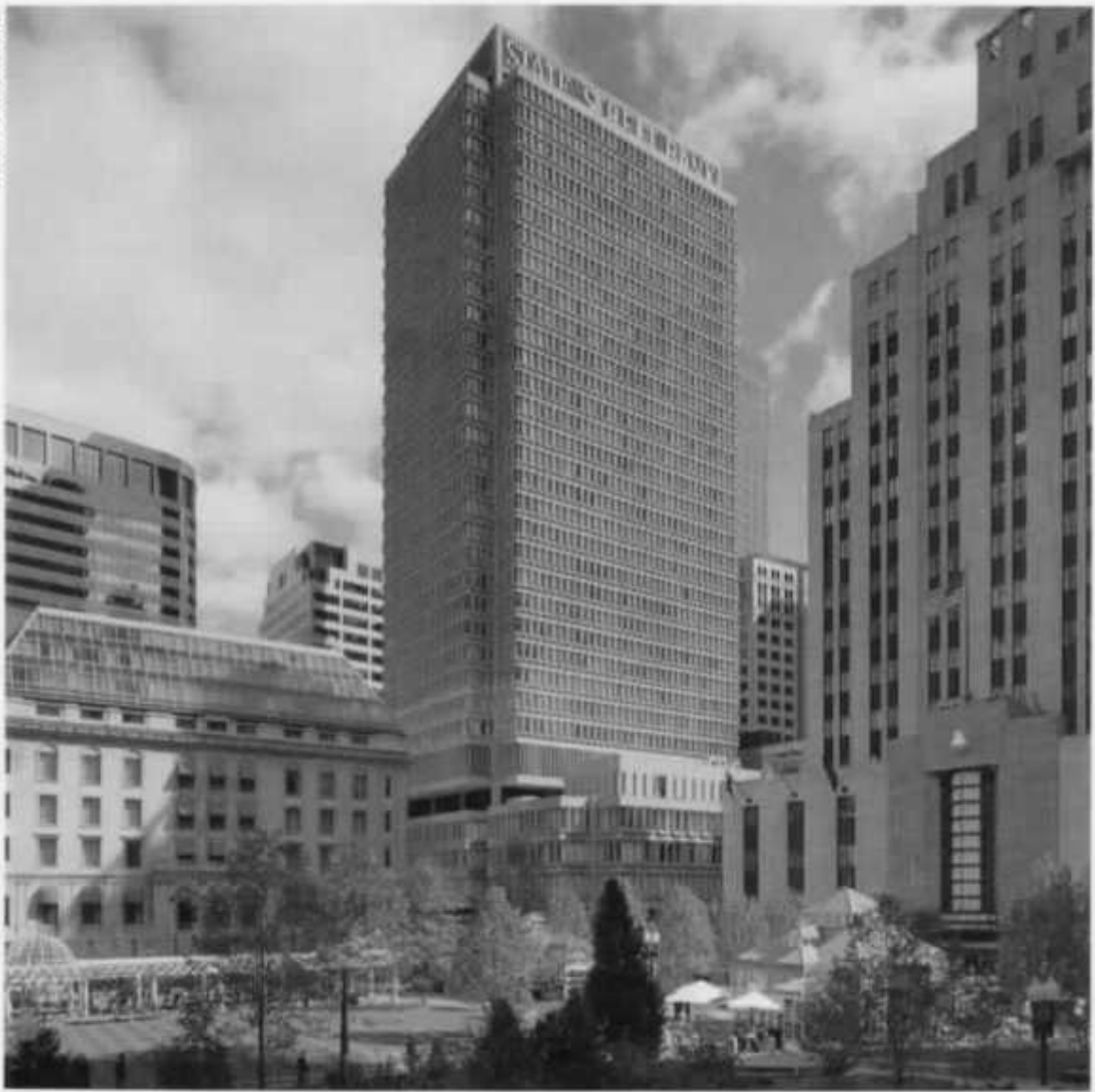
The newly renovated State Street Bank Building continues to be a landmark on the Boston skyline. Renovation dollars were spent where they would have the most impact—on the outside plaza, the lobby, the building systems, and asbestos abatement.
