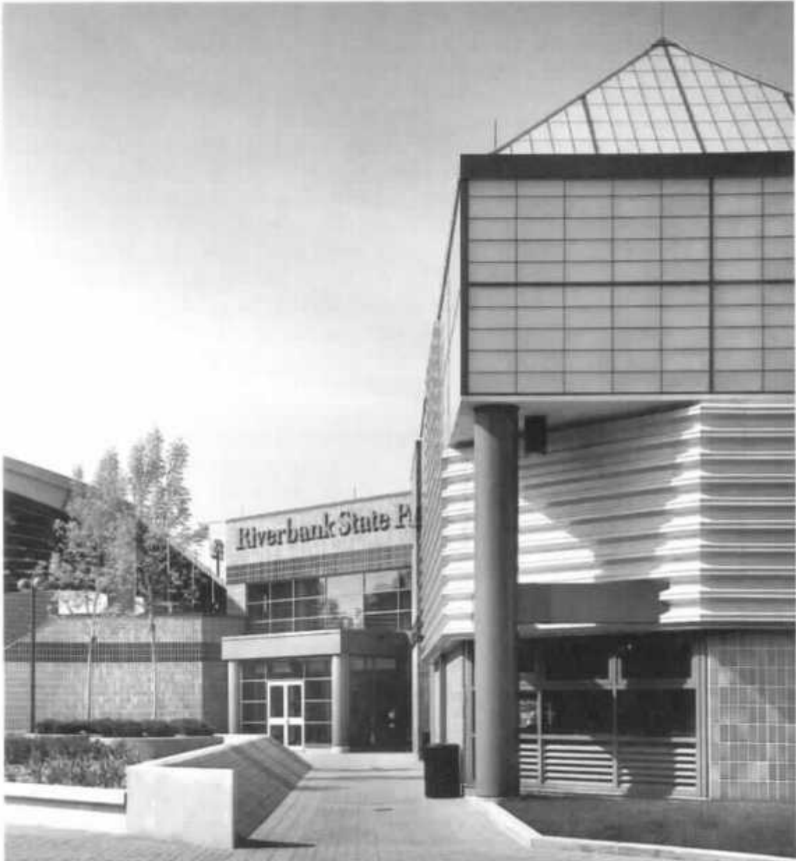
Building facades are wrapped in rust-colored brick tiles highlighted with a band of green, with red accents throughout. Fiberglass skylights cap four corners of all the buildings.
