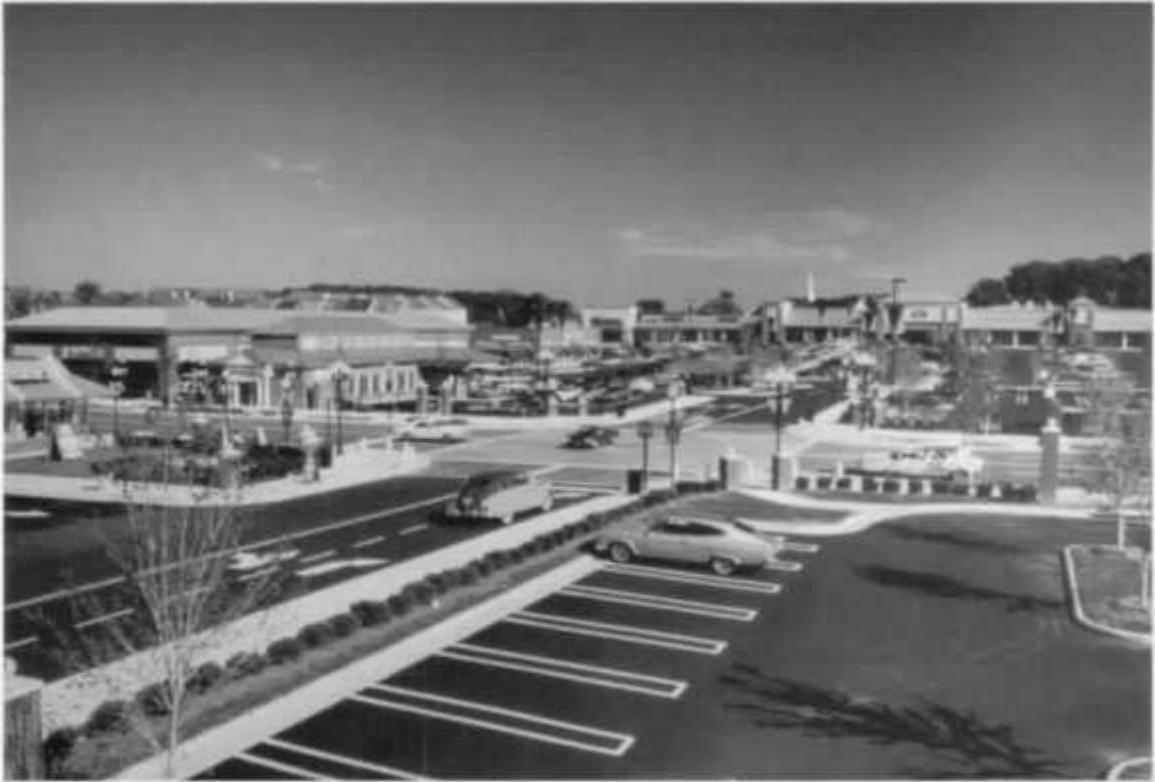
The complex features a neotraditional grid street layout. Grids were designed independently to ensure that regional destination shoppers did not interfere with community and neighborhood retail users.
