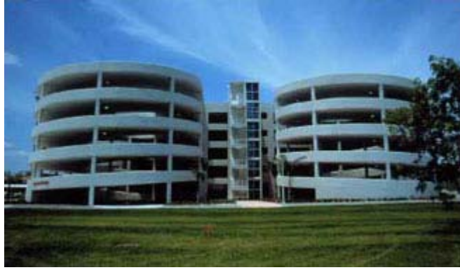
Two extrawide helixes vertically transport cars to open, level parking fields.
