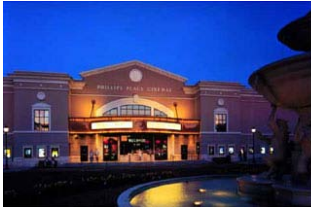
The phillips place Cinemas is a ten-plex movie theater with a state-of-the-art sound system and stadium seating coupled with the architecture of an old movie house.
