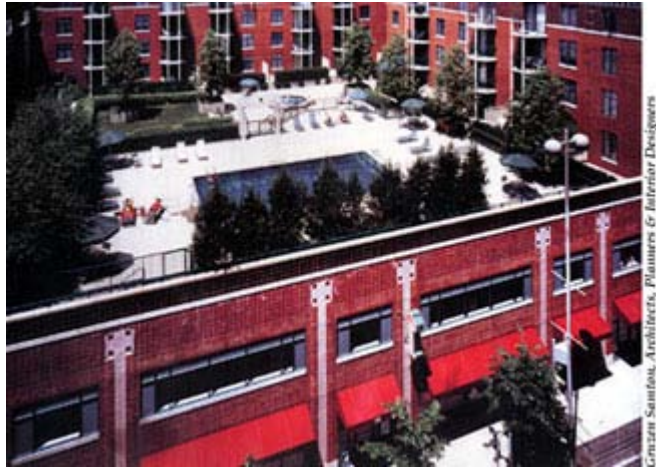
Residents of the Gramercy enjoy a landscaped courtyard with pool that sits on top of the building's parking garage. The windows visible on the second floor of the building help to disguise the parking garage.
