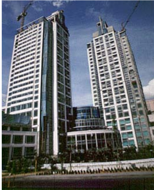
The new serviced apartment buildings under construction-the first in the philippines-articulate the entrance to Glorietta IV.
