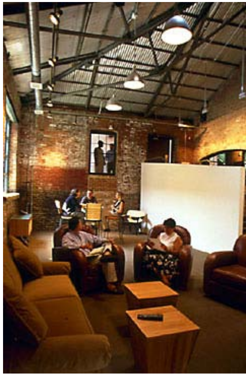
A 15-foot-wide slice was removed to create a skylit two-story atrium, bringing light into the interior and separating administrative and studio functions.
