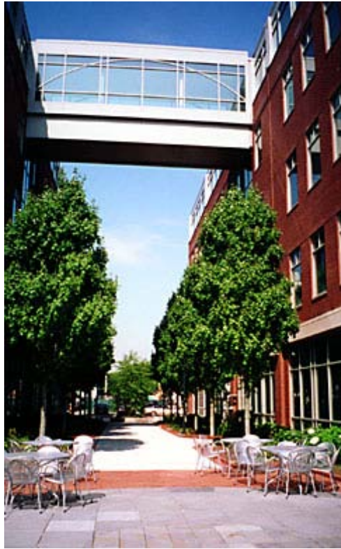
The bridge between the buildings was added during construction to provide a connection between two buildings with the same tenant. The vista under the bridge leads to the Auburn Court residential component and then into the adjacent community.
