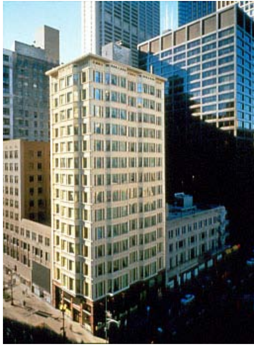
This view, taken from an identical vantage point as the previous image, shows how the surrounding downtown skyline has changed, while revealing how faithfully the city restored the building. Note the reconstructed cornice and the now-pristine terra-cotta cladding.
