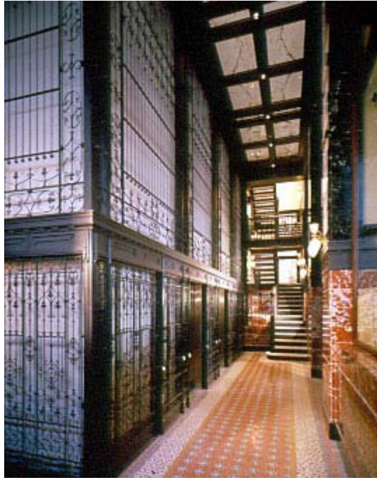
The elevator lobby uses original materials in a newly configured space: iron grillwork, mahogany paneling and trim at the walls and ceiling coffers, and a mosaic tile floor that leads past the elevators at left to a new monumental stairway that was extended down to the first floor from the historic seventh floor.
