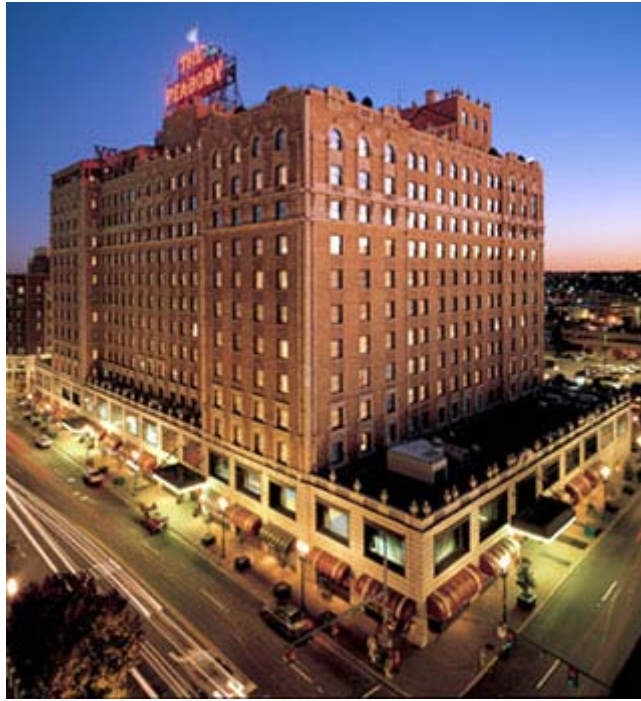
peabody Hotel. The 468-room peabody Hotel is a 14-story Italian Renaissance Revival building, built in 1925 during the era of the grand hotel. The masonry building has a terra-cotta and limestone base with terra-cotta cornices, pilasters, balustrades, and window surrounds on the upper levels.
