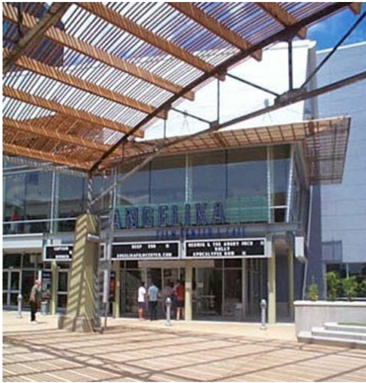
Angelika Film Center and Caf? is an eight-screen independent movie theater. RTKL designed a wood-latticed shade structure at the theater's entrance using steel trusses salvaged from elsewhere on the site.
