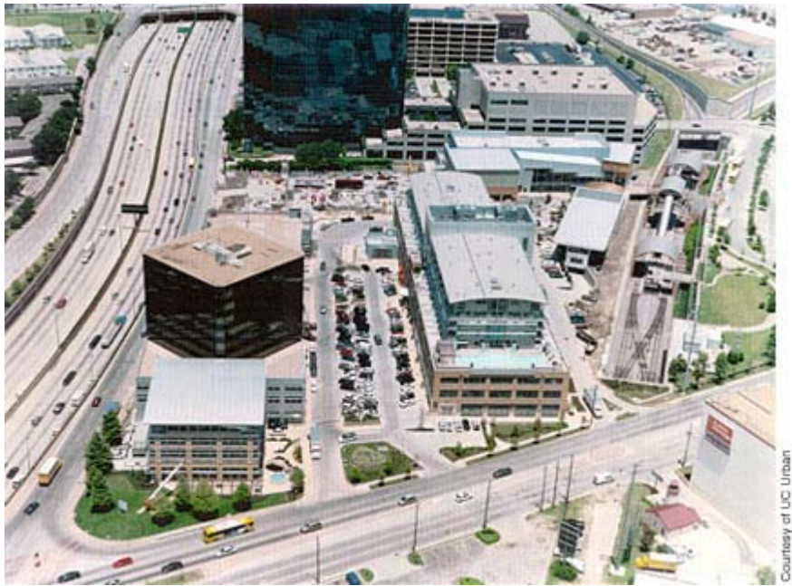
Aerial view of Mockingbird Station from the north.
