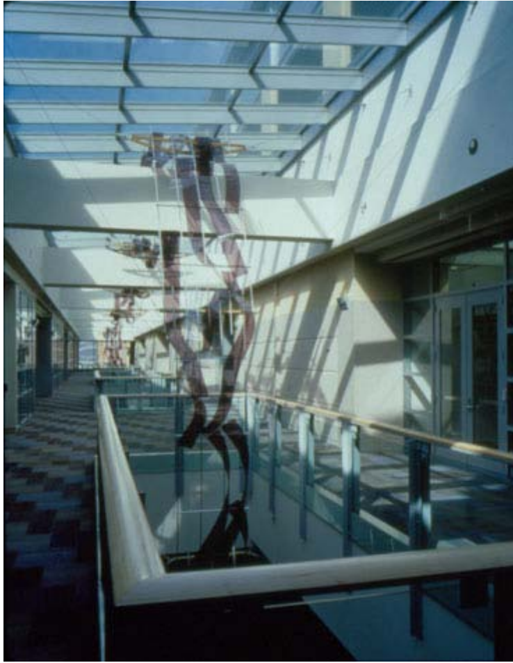
Views of light wells and skylights. Wide corridors with skylights and light wells that let in abundant daylight also facilitate circulation.
