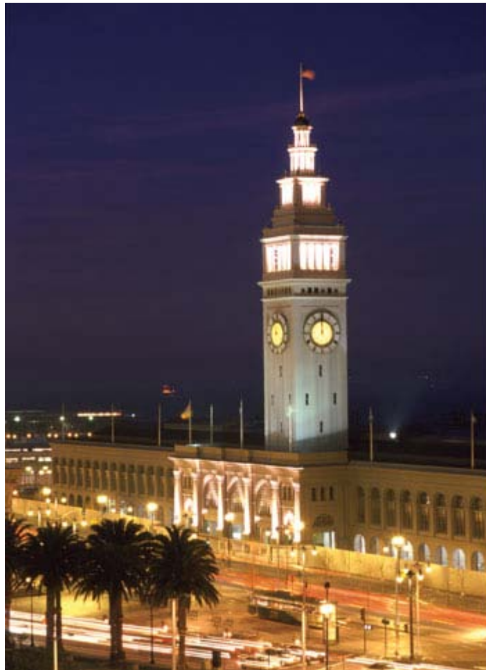
A four-year, $100 million restoration of the beaux arts Ferry Building on the San Francisco Bay. The 240-foot-tall clock tower, modeled after the bell tower in the Seville Cathedral, is a landmark on the waterfront.
