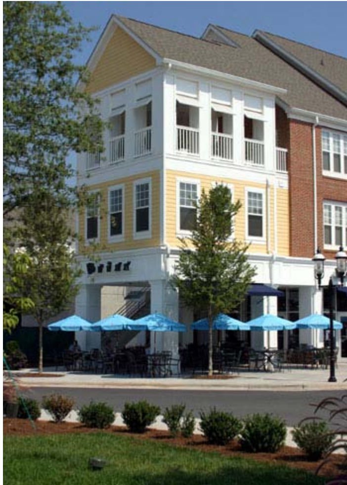
Clustering uses such as restaurants around the central green facilitates movement along the main street corridor.
