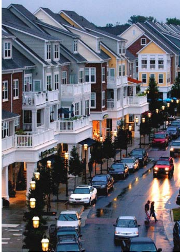
The location of residential units above main street retail creates an active urban village.
