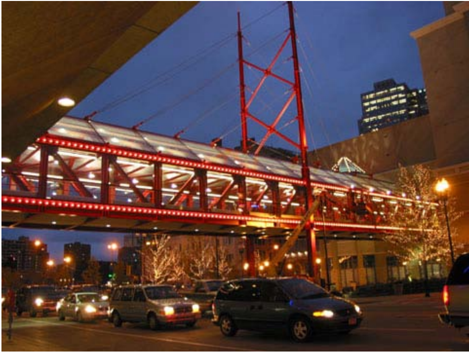
The skyway that connects Block E to the Target Center across First Avenue is the most dramatic in the city, with bold red coloring and soaring cables that resemble those of a suspension bridge.
