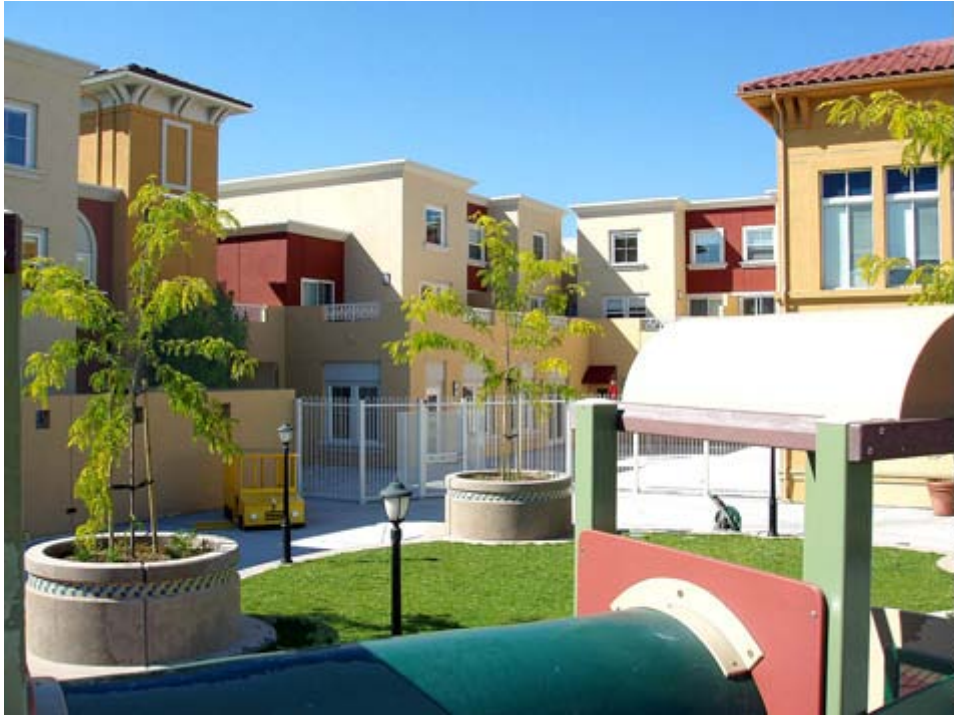
Both buildings in Fruitvale Village have outdoor patio spaces on their second levels that sit above covered parking garages (together the two structures provide 150 parking spaces). The southern building's patio features a play area for children enrolled in the Head Start program.
