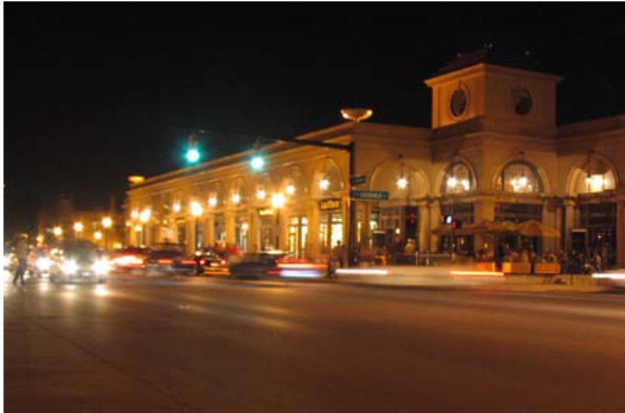
The Cap at Union Station is a $7.8 million retail development that reconnects downtown Columbus and its convention center with the burgeoning Short North arts and entertainment district.
