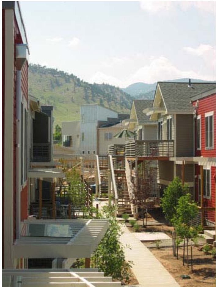
Consisting of three price-point levels, including four homes built by Habitat for Humanity, nine permanently affordable units, and 21 market-rate units, Wild Sage is a 34-unit, mixed-income, environmentally friendly cohousing project in Boulder, Colorado.
