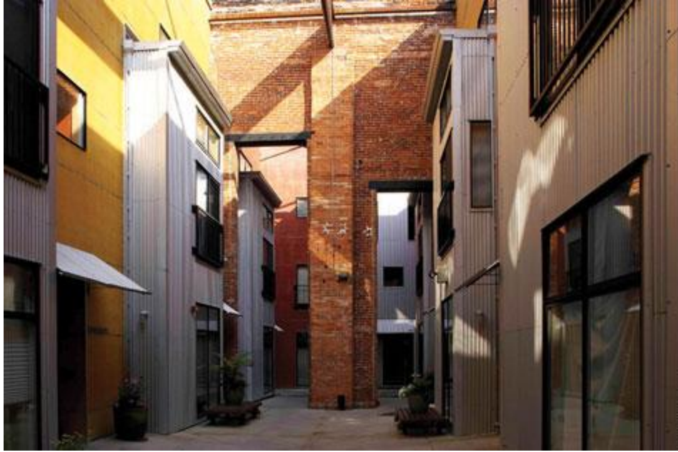
The developer reused the historic Cable Building, integrating the modern design of the new apartments with the brick masonry of the existing structure.
