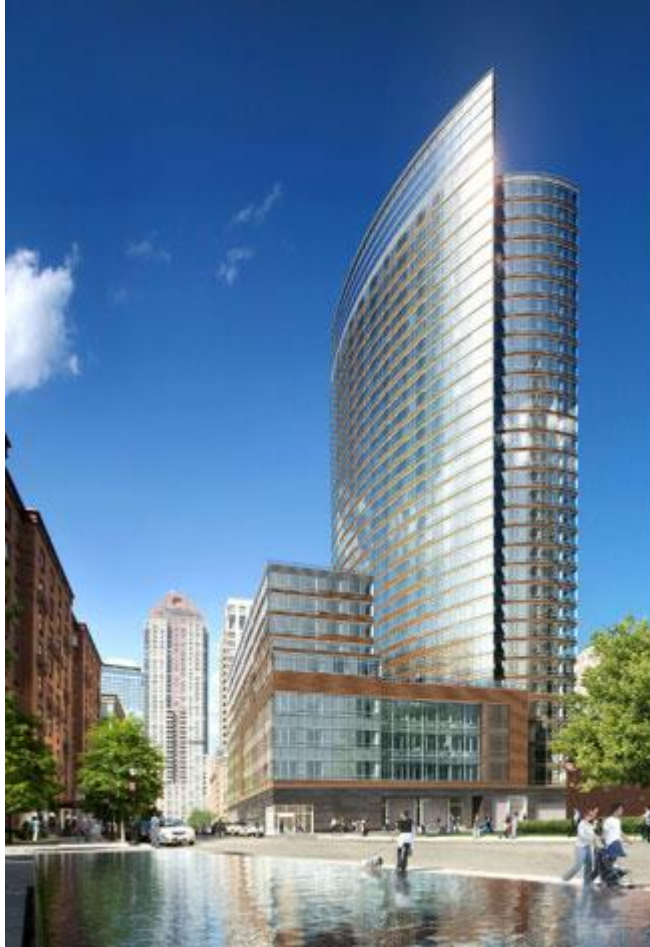
The Visionaire, located in New York City, is a 35-story, 537,400-square-foot (49,926-sq-m) condominium tower engineered to reduce energy consumption by 35 percent and achieve LEED Platinum certification.
