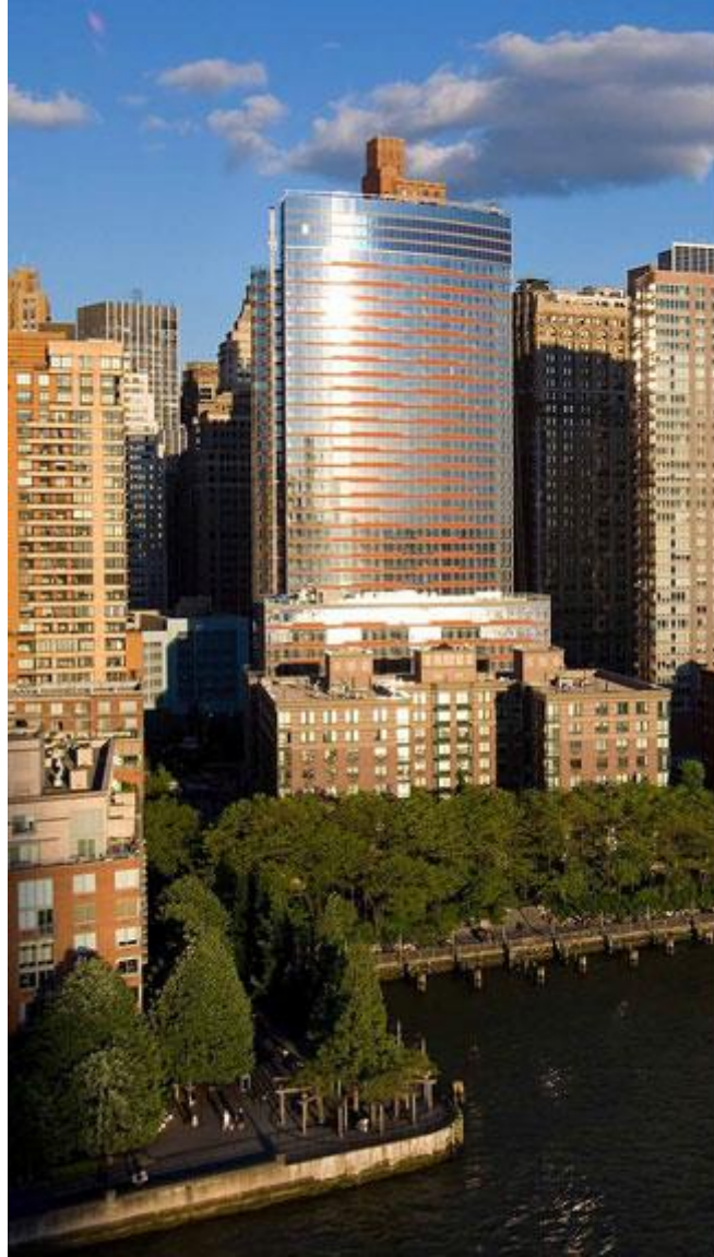
Situated in Battery Park City—a 92-acre (37.2-ha) master-planned community on the southwest corner of Manhattan Island—the 249-unit Visionaire was designed in compliance with stringent design and environmental guidelines.
