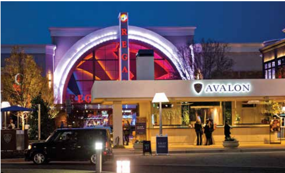
Avalon features a concierge desk at the center of the project—with a movie theater in the background—that provides hotel-style services for tenants and visitors alike.
