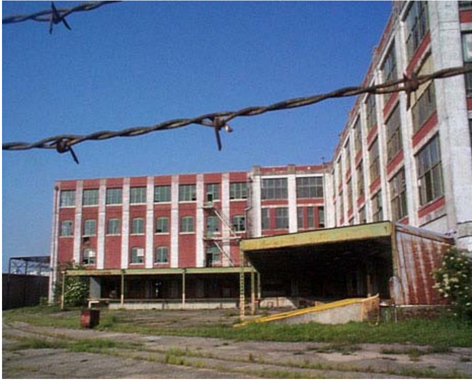
After the American Can Company plant closed in the 1980s, the complex sat empty and derelict for years.
