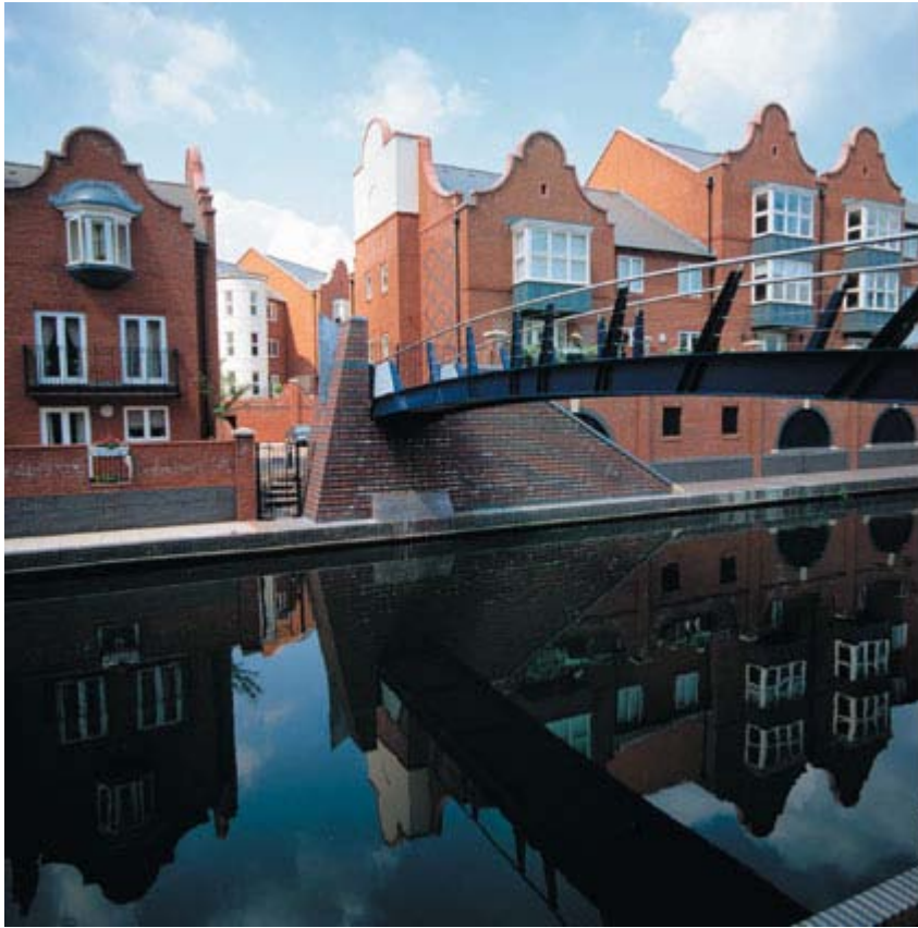
Set on a triangular site across from the Brindley Loop Canal, Symphony Court offers flats and townhouses with parking. The footbridge connects to Bridleyplace.
